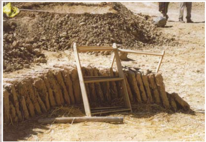
Wooden formers for bricks
