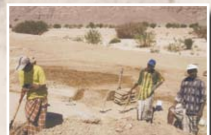
Digging out the footings for the school in Asnab
