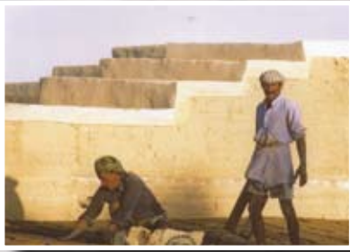
Bricklayers at work
