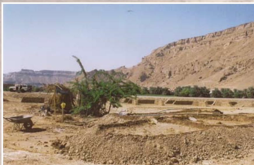
Puddling mud and straw for madar bricks and mortar
