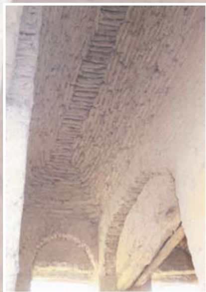
New corbelled vault in unfired mud-brick
